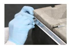
**Step 4**- Place the termination bar or strip aligned with the top of the PVC flashing
