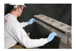
**Step 3**- Attach the PVC flashing to the wall. Continue the membrane down the wall, continue over the wall-to-footing transition and continue out to within 0.5" (1.27 cm) from the edge of the brick shelf.
