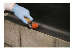
**Step 8**- Secure the PVC flashing to the brick shelf. Roll with a 1.5" (3.81 cm) roller to insure complete contact.
